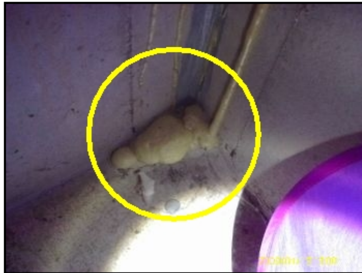
Repair to leaking foundation
