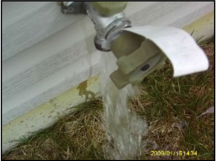
works - no leaks
