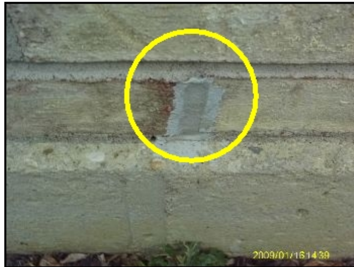
Repairs previously made
