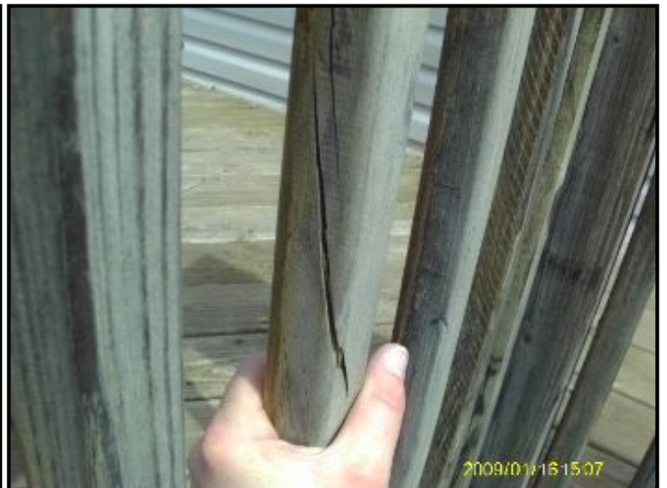
broken baluster
