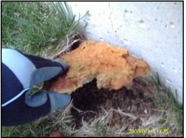
Piece of insulation against foundation
