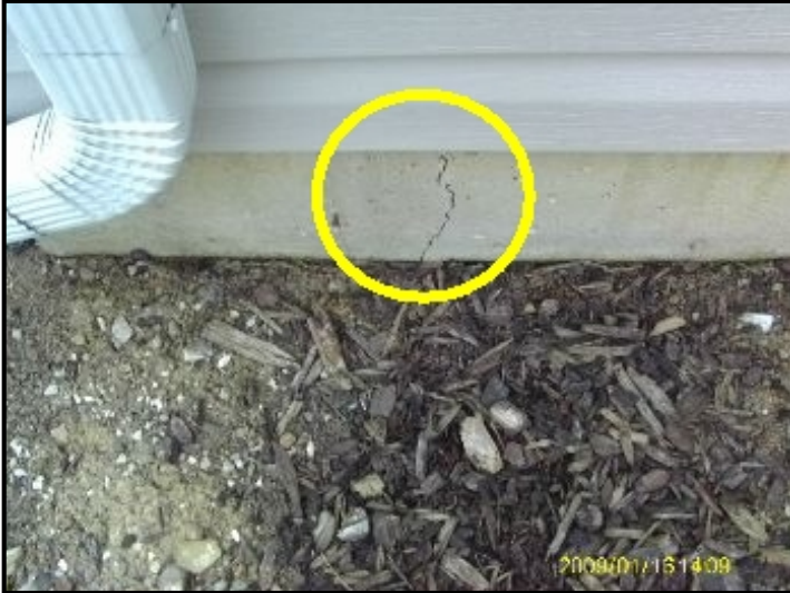
Vertical Crack
