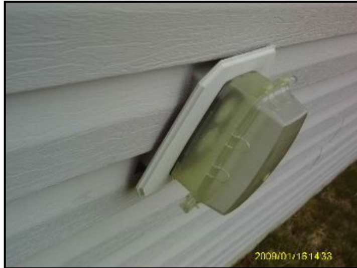
Unit not flush with wall
