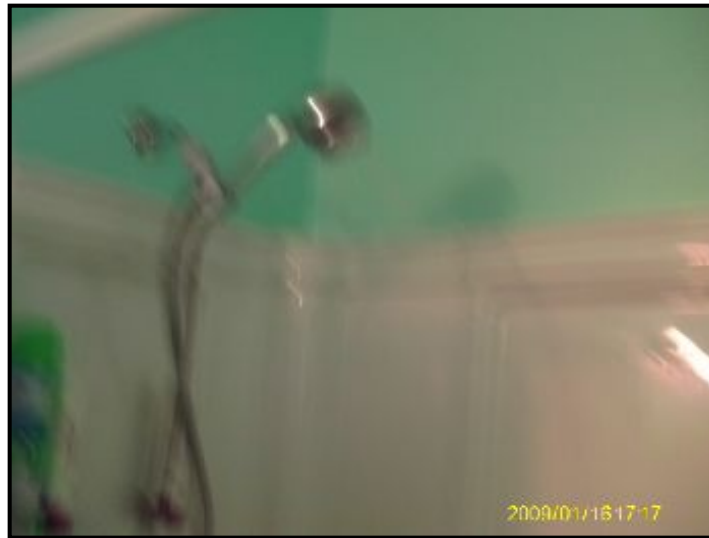
Master Bathroom shower is functional
