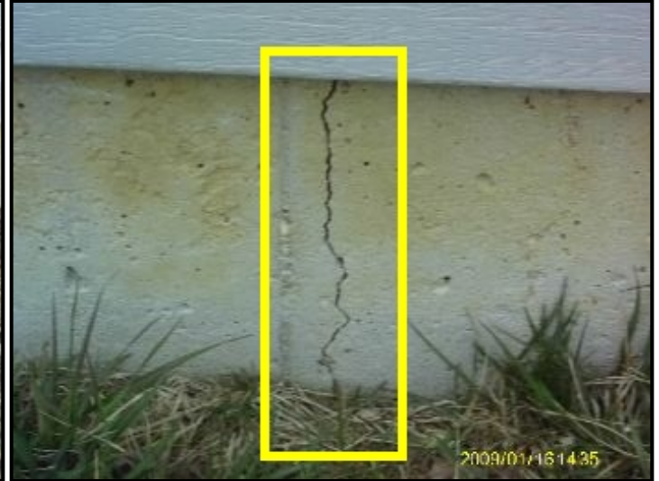
Vertical Crack
